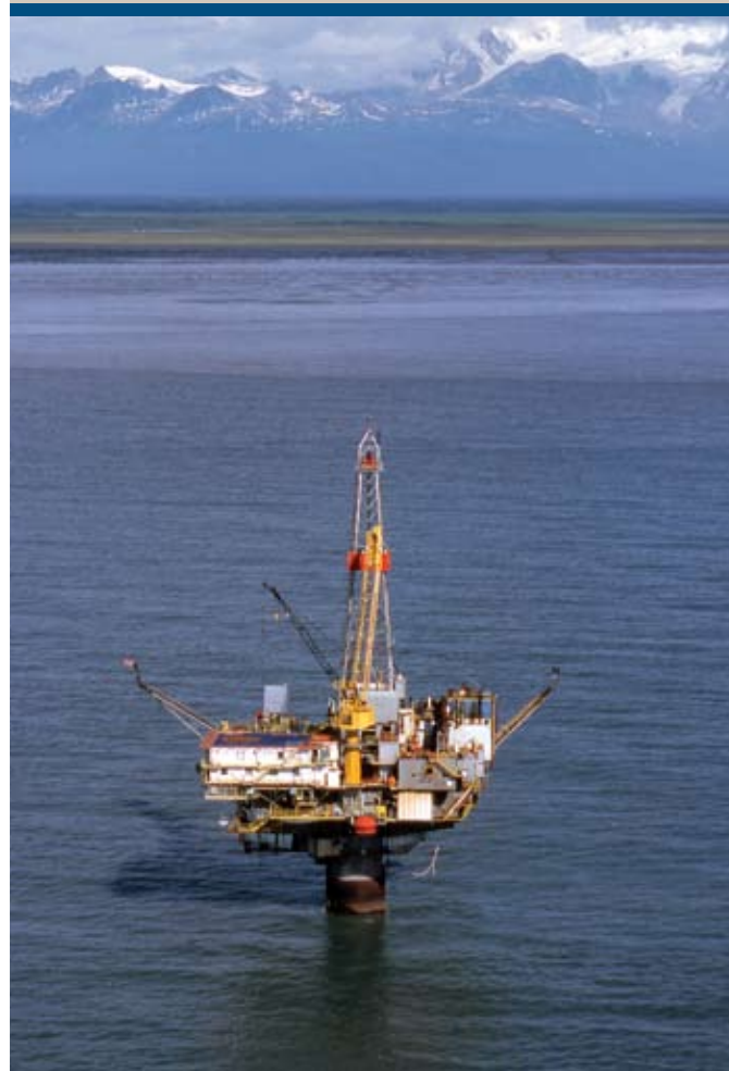
Chevron’s monopod platform located in Cook Inlet.
